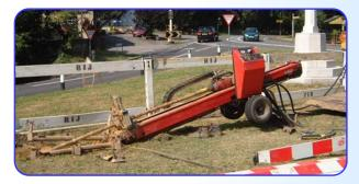
We employ the latest trenchless installation techniques to simplify the process of installing pumped rising mains, water pipes, gas pipes and service ducts whilst minimising disruption and greatly reducing reinstatement costs.
