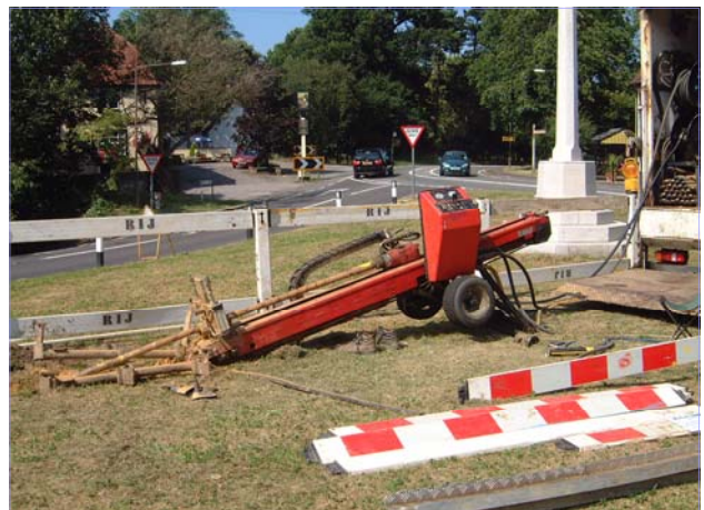
Trenchless Installation of the pumped rising main
