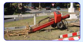
We employ the latest trenchless installation techniques to simplify the process of installing pumped rising mains, water pipes, gas pipes and service ducts whilst minimising disruption and greatly reducing reinstatement costs.
